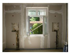
Analyzed room with opened areas for the installation of the sensors.
