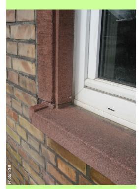
Insulated window frame at the same position. Reduction of thermal bridges by connecting the interior insulation (see page 5)
