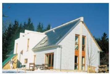
• To reach high fractional-energysavings, huge collectors have to be installed, Two-family house, House Schiretz, Hitzendorf, AEE INTEC, Austria
