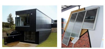
Figure 1: Left: Scalable, facade integrated polymeric collectors (source: Aventa) Right: Scalability illustrated at the SHC2013 (Fraunhofer ISE).
