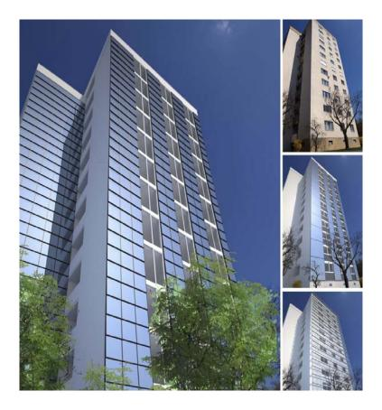
Figure 6: Alternative approaches for integrating solar thermal collectors into high rise apartment building from the late 1960 in the course of a renovation study, Source: Institute of Architectural Typologies, Graz Technical University
