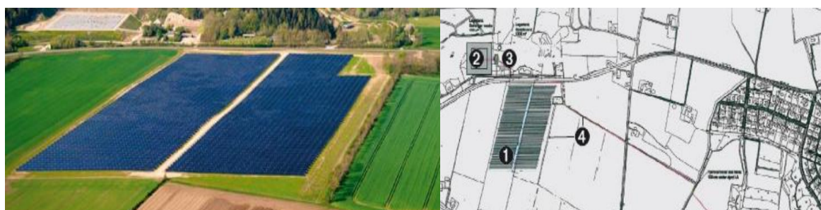
Figure 17. Overview over the collector field in Dronninglund (left) and schematic over the different components (right) where the collector field (1) is constructed next to the pit storage (2) and solar central (3). The DH pipes (4) closely follow the right side of the collector field.
