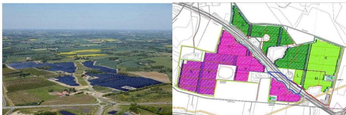
Figure 1. Overview over the installation in Silkeborg (left) and schematic showing the different sections and piping of the installation. (right). Source: Silkeborg Forsyning AB
