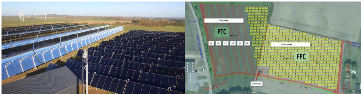
Figure 12. Overview over the installation in Taars (left) and schematic showing the different sections of the installation (right).
