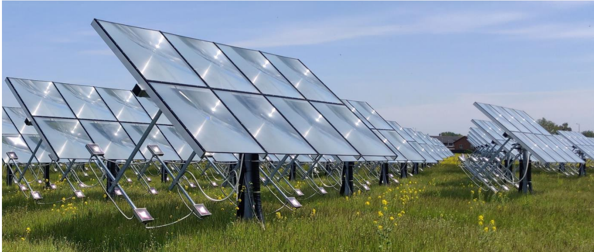
Figure 24 Photo of Fresnel lenses, Heliac in Denmark (Jensen, Sifnaios, Caringal, Furbo, Dragsted, 2022)
