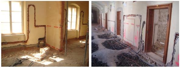
Pipe distribution in the corridor of the monastery for the component low-temperature heating (AEE INTEC)
