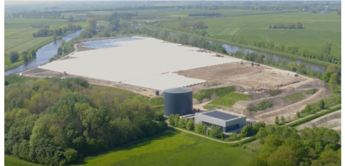
Photo: TVP Solar from Video of the construction site: https://www.youtube.com/watch?v=WfwXdOkpHkY&t=4s
