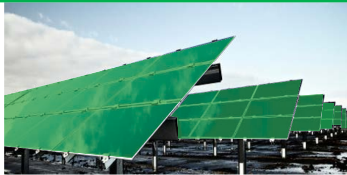
Figure 5 - The photovoltaic space [6] (Source: © Enbridge Inc.)
