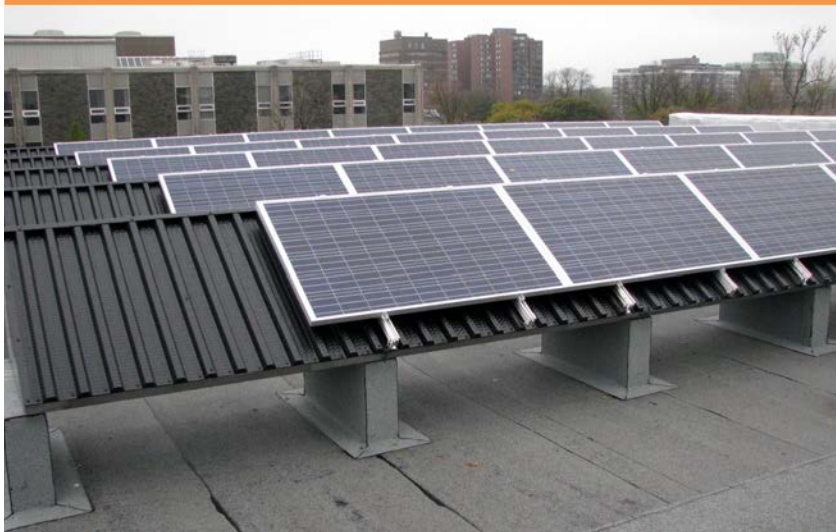
Figure 5 - Solar PV on the roof of the room of the Goldberg Computer Science Building.. (Photo: © Dalhousie University )
