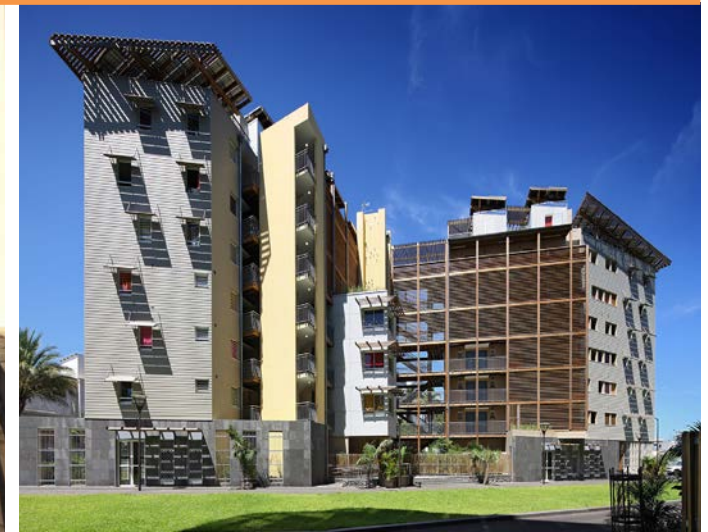
Figure 15 - Solar protection is the key in the tropical climate of Reunion Island. Optimised solar shading devices, over-roofs and external passageways are architecturally integrated in the Flores Malacca project. (Photo: © H. Douris)
