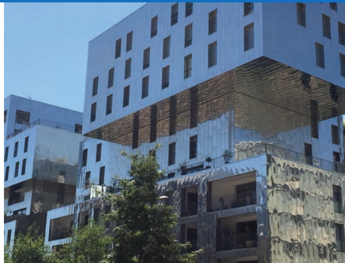
Figure 16 - Stainless steel building envelope. (Photo: © C.Ménézo)
