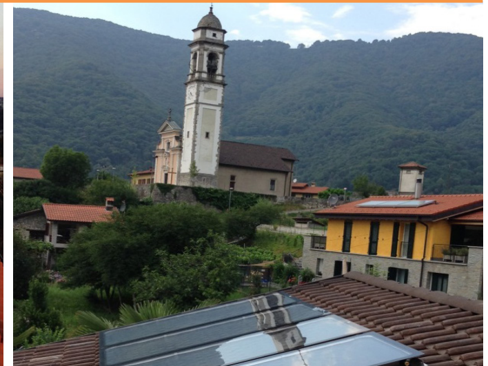
Figure 18 - New solar thermal installation. (Source: © SUPSI)
