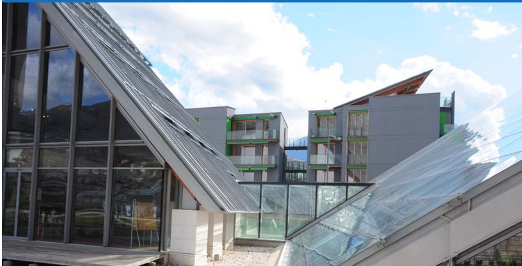
Figure 15 - On the front: the MuSe and its greenhouse; on the back: the buildings of the residential-commercial district. (Photo: © Silvia Croce)
