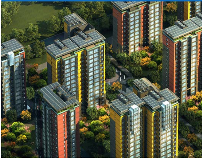
Figure 1 - Schematic layout of roofing system for solar collector arrangement (Source: © Beijing Institute of Residential Building Design & Research Co., Ltd, 2011.)
