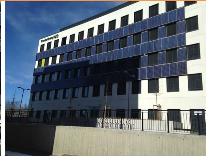
Figure 6 - South view of the BiPV facade of the office building in Trondheim, Norway. (Photo: © Carmel Lindkvist)
