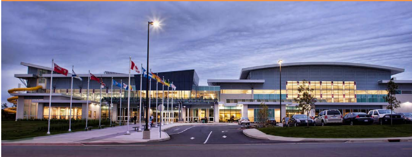
Figure 1 - A view of the Halifax Canada Games Centre with photovoltaic panels installed on the roof of the building. (Source: © Canada Games Centre)
