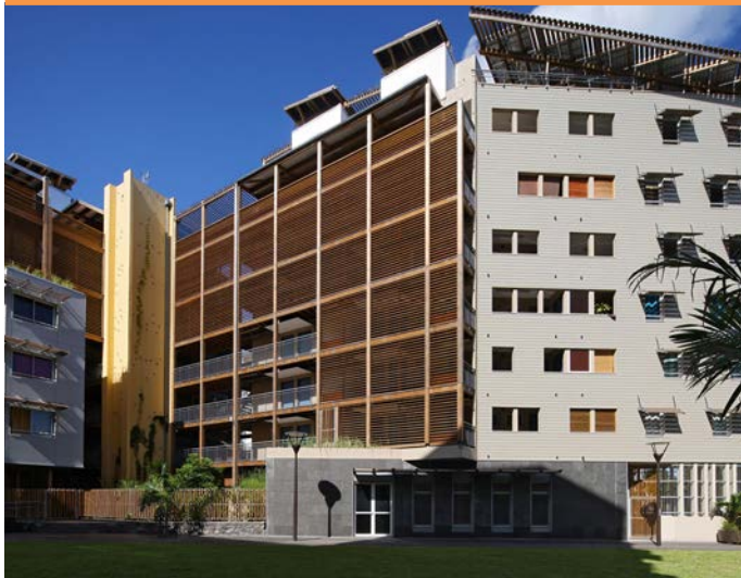
Figure 13 - The vegetated buildings' surroundings that contribute to cooling the atmosphere by evapotranspiration are watered with the rain and grey water collected on site. (Photo: © H. Douris)
