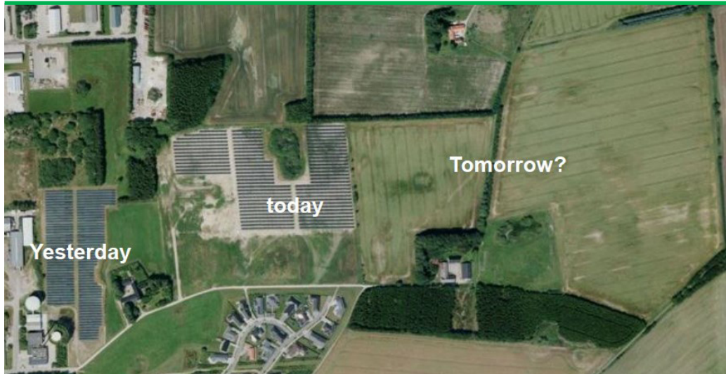
Figure 7 - Aerial view of the total area: Stage 1 and 2 ("Yesterday" and "today") and the potential stage 3 ("Tomorrow?") showing the vision for a future expansion of the solar thermal plant. (Source: © Municipality of Horsens)
