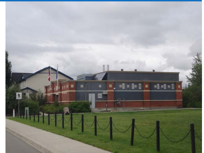
Figure 13 - Borehole field (foreground) and Energy Centre after construction (Photo: © N.Robertson, 2016)
