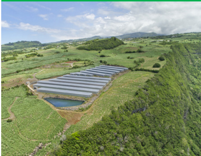
Figure 1 - Aerial view of the Agrinerjie 5 from the South. (Source: © akuoenergy)
