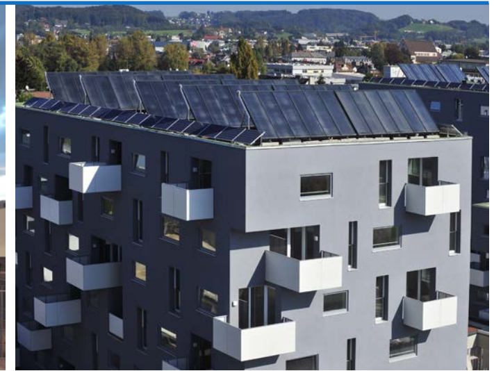
Figure 3 - Residential building with 2.000 m 2 of solar thermal collectors and 50 kWp PV on the roofs. (Photo: ©Fotohof Phelps)
