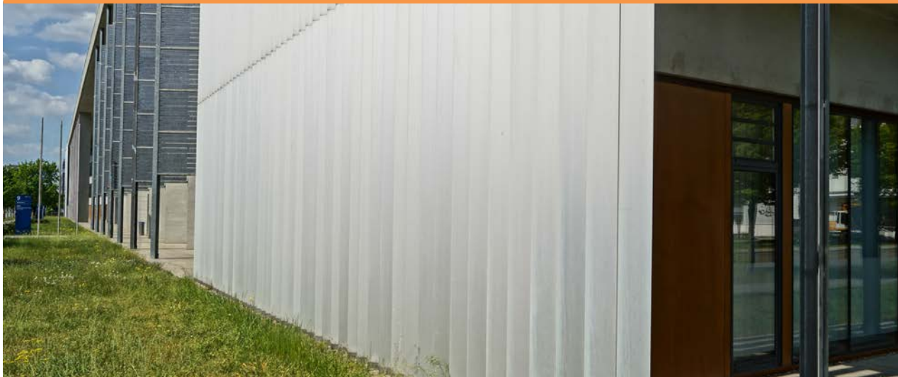
Figure 21 - Centre of Biotechnology and the Environment (Photo: © Margarethe Korolkow)
