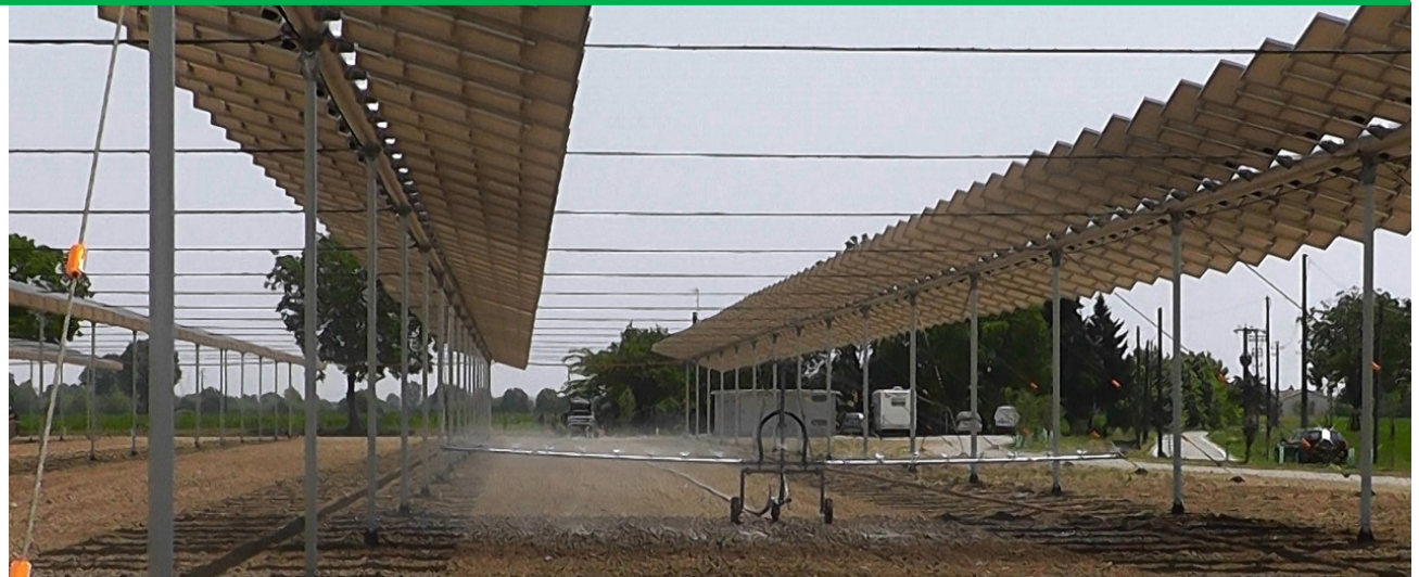
Figure 9 - Irrigation system in action under the PV track system. (Photo: © REM)
