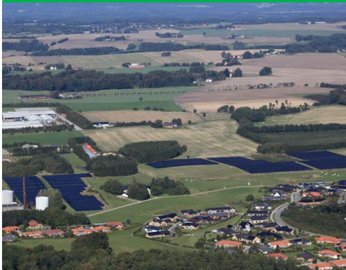
Figure 1 - Aerial view of the solar plant in landscape next to the town of Brødstrup. (Photo: © Brødstrup Fjernvarme)
