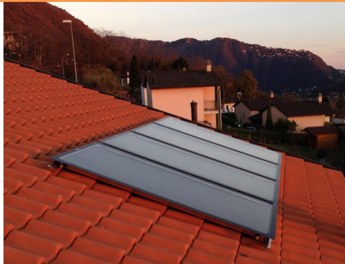
Figure 17 - New solar thermal installation. (Source: © SUPSI)
