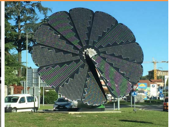
Figure 20 - Example of BIPV integration in an urban furniture element, Chiasso, Tessin Canton (CH) developed by Agere SA. (Photo: © Cristina Polo).
