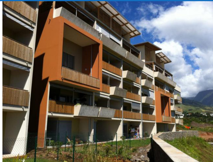
Figure 6 - Buildings integrate traditional creole porches and large roof overhangs to protect the buildings from adverse solar heat gains. (Source: © H. Douris)
