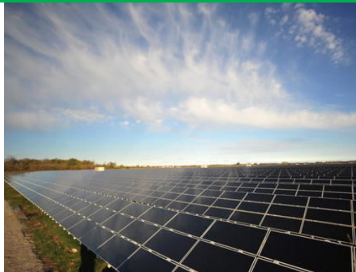
Figure 8 - Solar Panels. (Source: © Postmedia Network)
