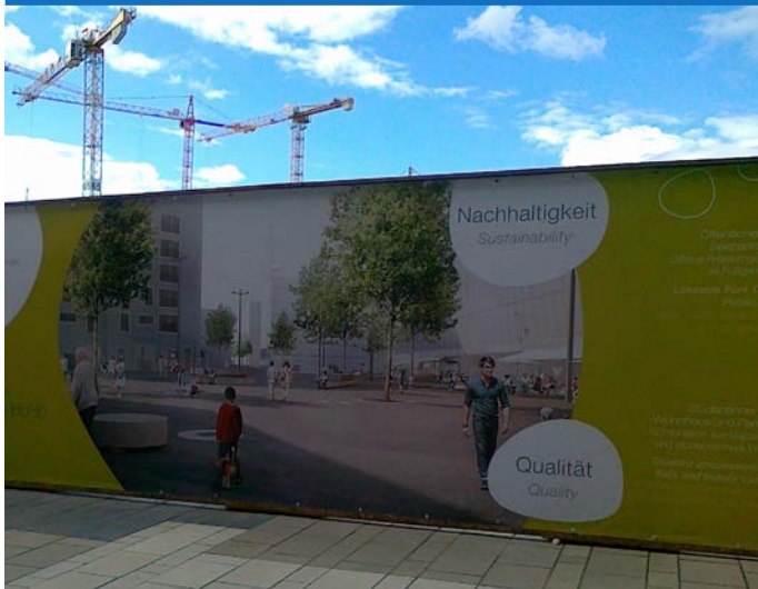
Figure 8 - Aspern under construction (Photo: ©Daiva Jakutyte-Walangitang)
