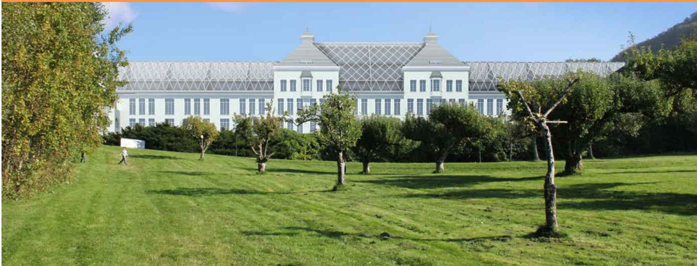
Figure 5 - East view of the refurbishment intervention of the main building of Dale (Source: © KOKO architects, 2014)
