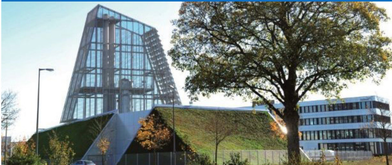
Figure 5 - Chimney of the heating plant of Freiham, including PV modules. (Photo: © Stadtwerke München)
