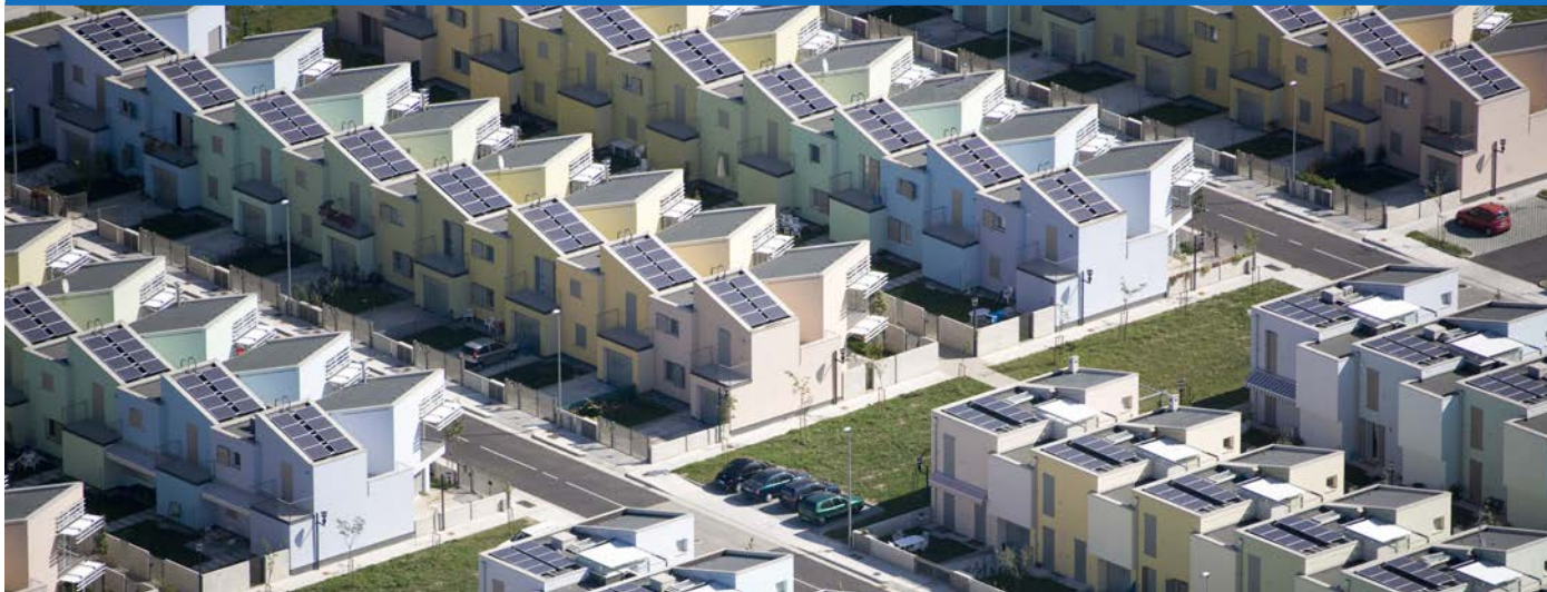
Figure 5 - Aerial view of the BiPV system on the roof of the 112 terraced houses (Source: © BAMSphoto - Basilio)
