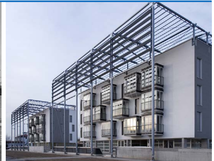
Figure 12 - South Side of the two multifamily houses. (Photo: © Fabio Cattabiani).
