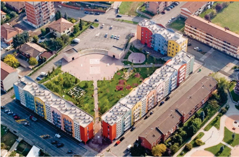
Figure 1 - Aerial view of the eastern area of the Photovoltaic Village. (Source: © Municipality of Alessandria)
