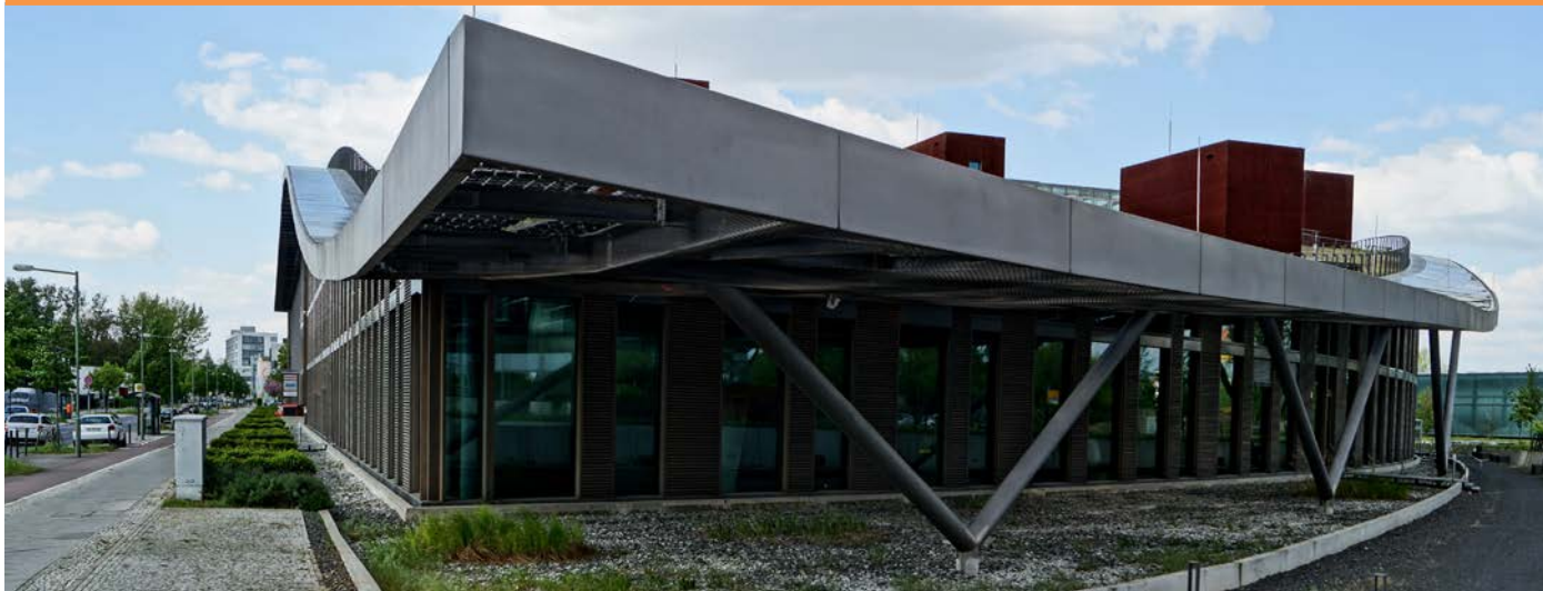
Figure 11 - Solon Headquarters (Photo: © Margarethe Korolkow)
