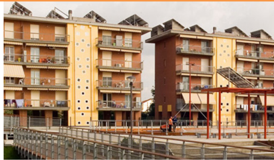
Figure 4 - PV panels installed on over-roofs on the row houses of the district. (Source: © A4 - Architettura Integrata)
