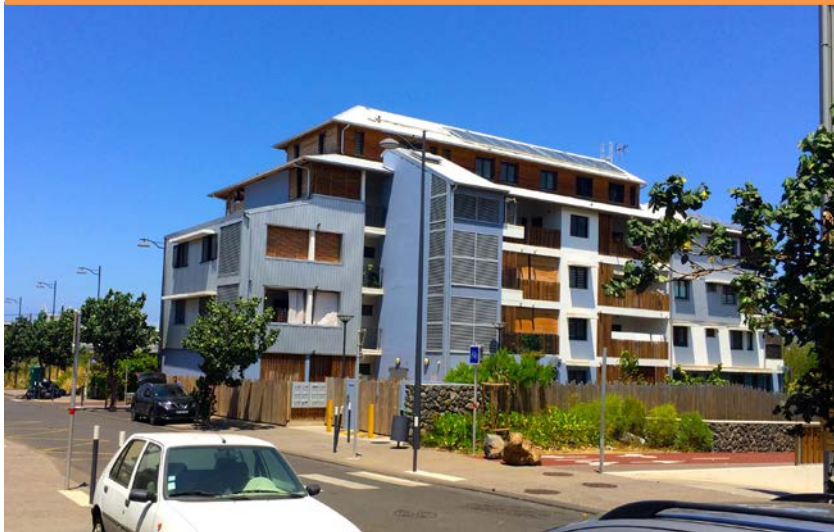
Figure 8 - Various solar shading devices, optimized according to the orientation of the facades, protect the numerous openings. (Source: © City of Saint-Pierre).
