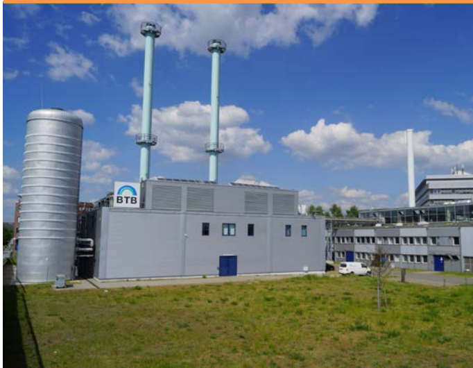
Figure 5 - Heating power plant with storage tanks and PV system. (Photo: © Margarethe Korolkow)
