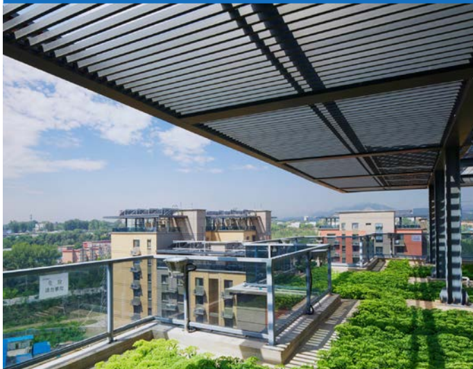
Figure 10 - View of green roof. (Source: © www.zhulong.com)
