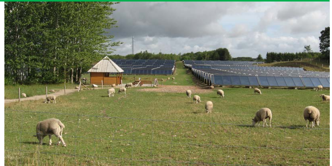
Figure 9 - View of the actual visual impact of the first stage in the project including integration of a wooden pavilion built to invite local citizens to visit the area. (Source: © Brædstrup Fjernvarme)
