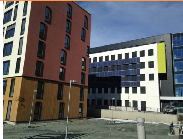
Figure 10 - A view of PV system installed on the South façade of the building. The PV panels resulted partly covered by the shadowing of the new student block built one year later. (Photo: © Carmel Lindkvist)
