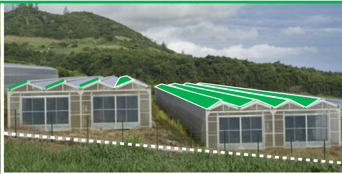
Figure 6 - The photovoltaic space (Source: [2])
