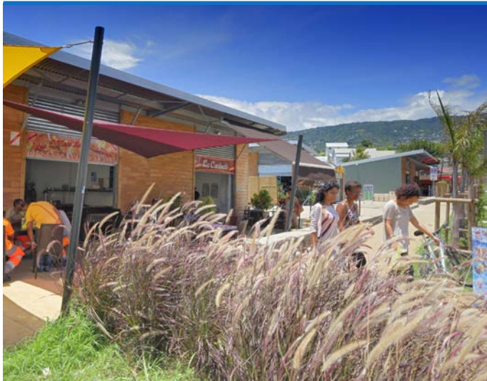
Figure 14 - Temporary shops were built early 2013 to provide services to the first inhabitants of the district. (Photo: © Tekhnê Architectes)
