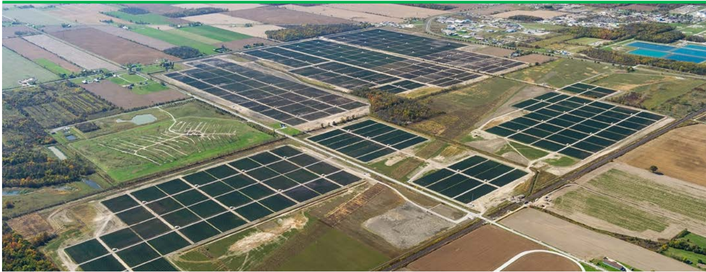
Figure 9 - Aerial view of the Sarnia Solar Project (Photo: © Daniel J Bellyk)
