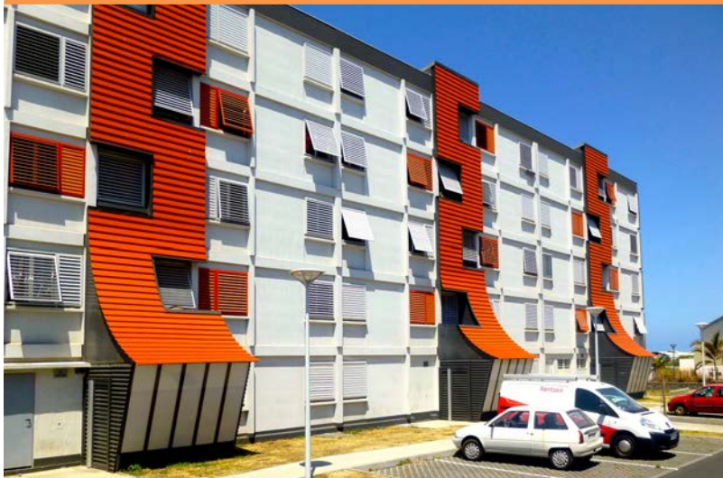
Figure 5 - Different passive design strategies have been implemented in order to reduce energy consumption while maintaining satisfactory thermal comfort conditions inside the buildings. (Source: © T. Giraud / City of Saint-Pierre)
