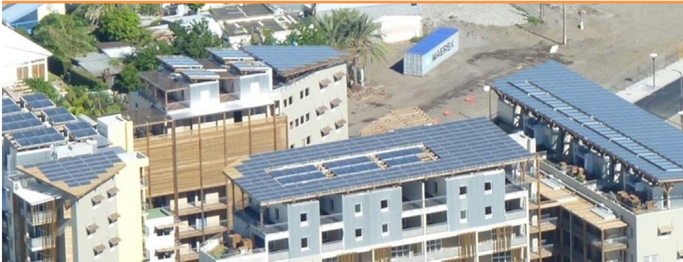
Figure 6 - System geometry [3]. Overview of the combined PV and solar thermal panels roof plant. (Source: © AP Architectures/2APMR)
