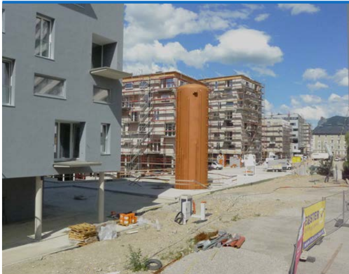
Figure 1 - Heat storage (200.000 l) during construction. (Photo: ©SIR Strassl)
