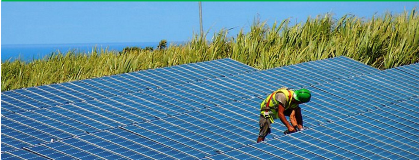
Figure 8 - View of the solar panels on the roof of the greenhouse space (Source: © akuoenergy)
