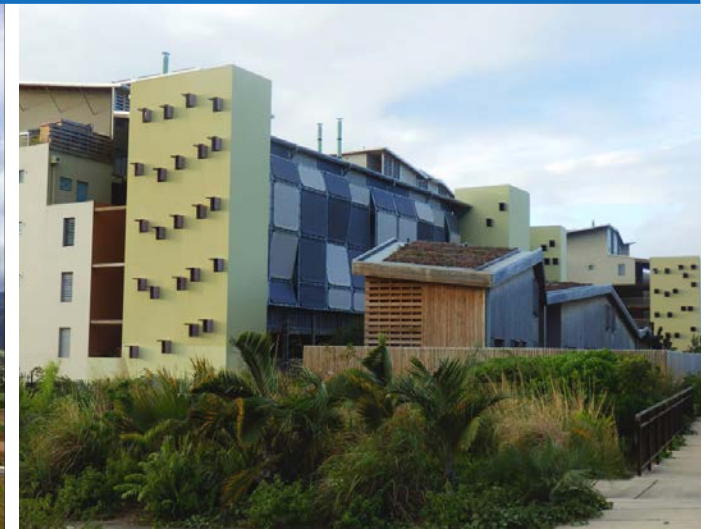
Figure 7 - The Portes de Beausejour apartment buildings are cooled by evapotranspiration and cross ventilation. Venturi-effect wind generators ensure the ventilation of bathrooms and kitchens. (Source: © JLU- Julien Lebreton).
