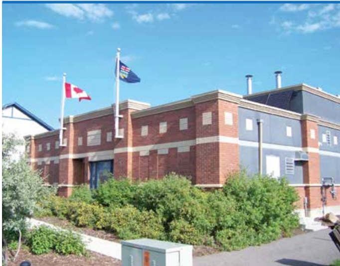
Figure 1 - Energy Centre (Source: © CanmetENERGY, Natural Resources Canada)
