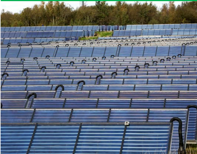
Figure 11 - View of solar collectors in the first stage of the project. (Photo: © Brædstrup Fjernvarme)
