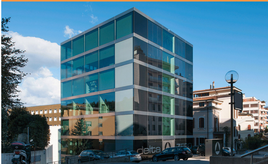
Figure 10 - View of the deltaZERO building (Source: © deltaZERO deAngelis Mazza and associates)
