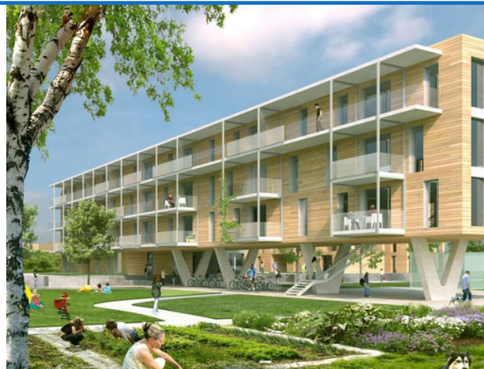
Figure 9 - Social housing (Quarter 8) at the southern part of Reininghaus. (Source: Nussmüller Architekten ZT GmbH)
