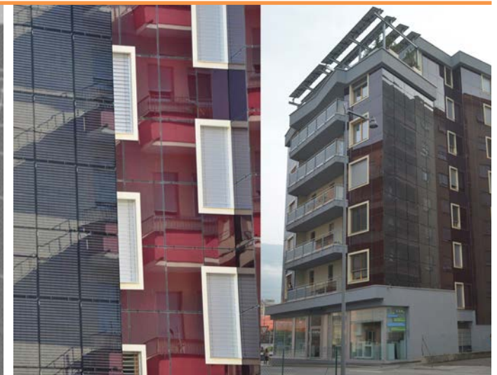
Figure 13 - Example of complete BIPV façade and roof integration in an urban existing environment: Palazzo Positivo Gasser residential renovated building, Chiasso, Tessin Canton (CH). Plus Energy House and Swiss Solar Award 2014. (Source: © ISAAC-SUPSI)
