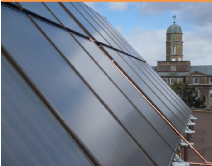
Figure 3 - Solar Water heating at Dalhousie Life Science Center. (Source: © Halifax Regional Municipality)
