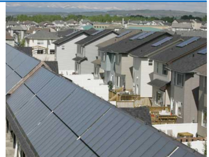
Figure 8 - Modular pattern. View of ST collectors on garage roofs (foreground) and DHW panels on homes. (Source: © CanmetENERGY, Natural Resources Canada) [8]
