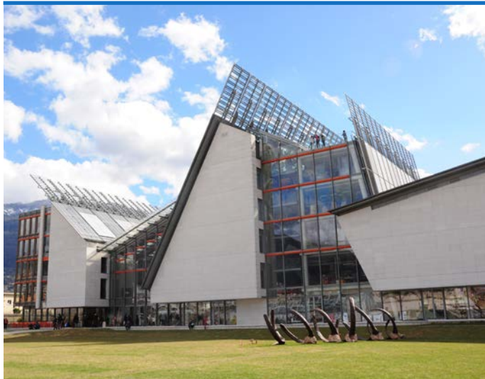
Figure 8 - North view of the science museum MuSe. The PV are integrated in the top surfaces of the roofs (Photo: © Silvia Croce).
