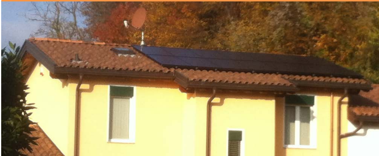
Figure 9 - View of PV panels installed on the roof. (Source: © SUPSI)
