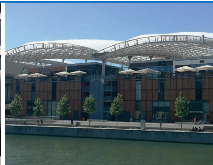
Figure 2 - Commercial Buildings of phase 1. (Photo: © C. Ménézo)
