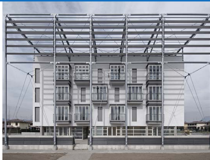
Figure 2 - Southern façade of the multifamily house. (Photo: © Fabio Cattabiani)
