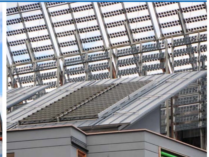
Figure 5 - The two typologies of BiPV systems: Tedlar-glass modules on the zinc roof and glass-glass modules (Photo: © Silvia Croce).
