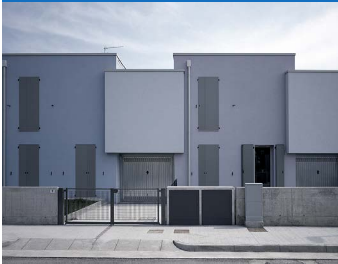
Figure 17 - West side of the terraced house. (Photo: © Alberto Mucciaccia)
