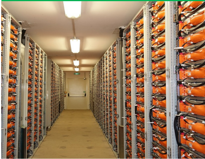
Figure 1 - Inside view of battery system integrated in containers (Source: © akuoenergy.com)
