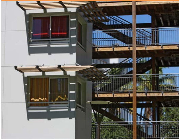
Figure 10 - The presence of wooden elements is marked on the project: from the structure of the over-roofs and passageways to solar shading blades. (Photo: © H. Douris)
