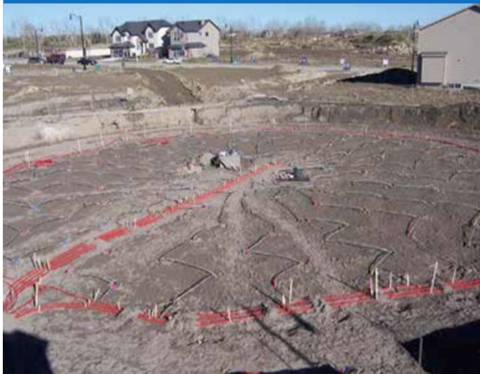
Figure 11- Borehole field under construction (Source: © CanmetENERGY, Natural Resources Canada)
