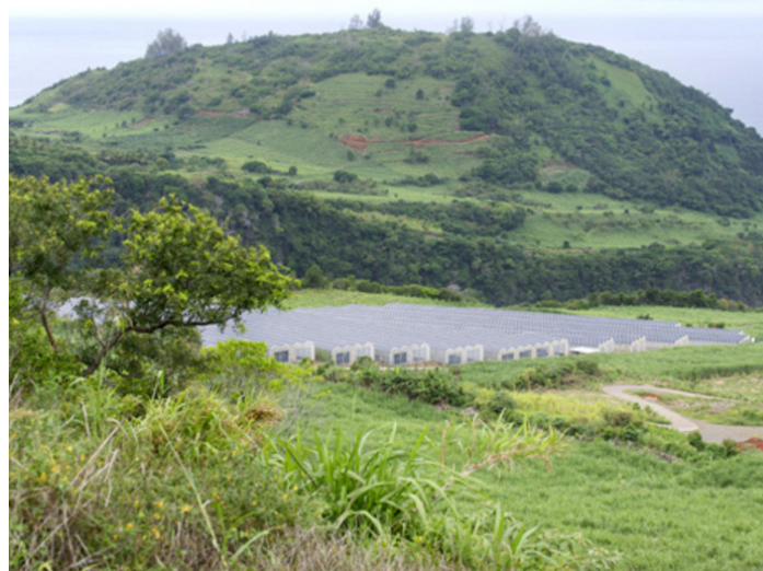
Figure 2 - View of the PV system integrated in the roof of the greenhouses from the North. (Source: © akuoenergy)
