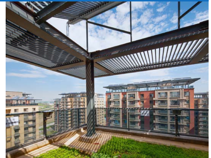
Figure 15 - View of green roof. (Source: © www.zhulong.com)
