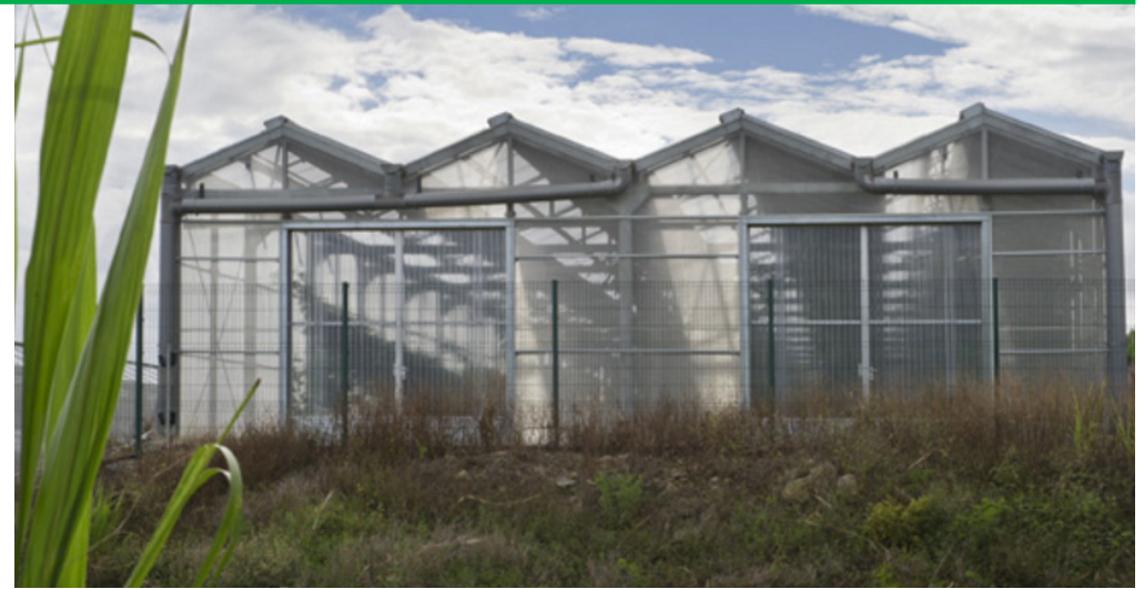
Figure 13 - View of the greenhouses (Source: © akuoenergy)
