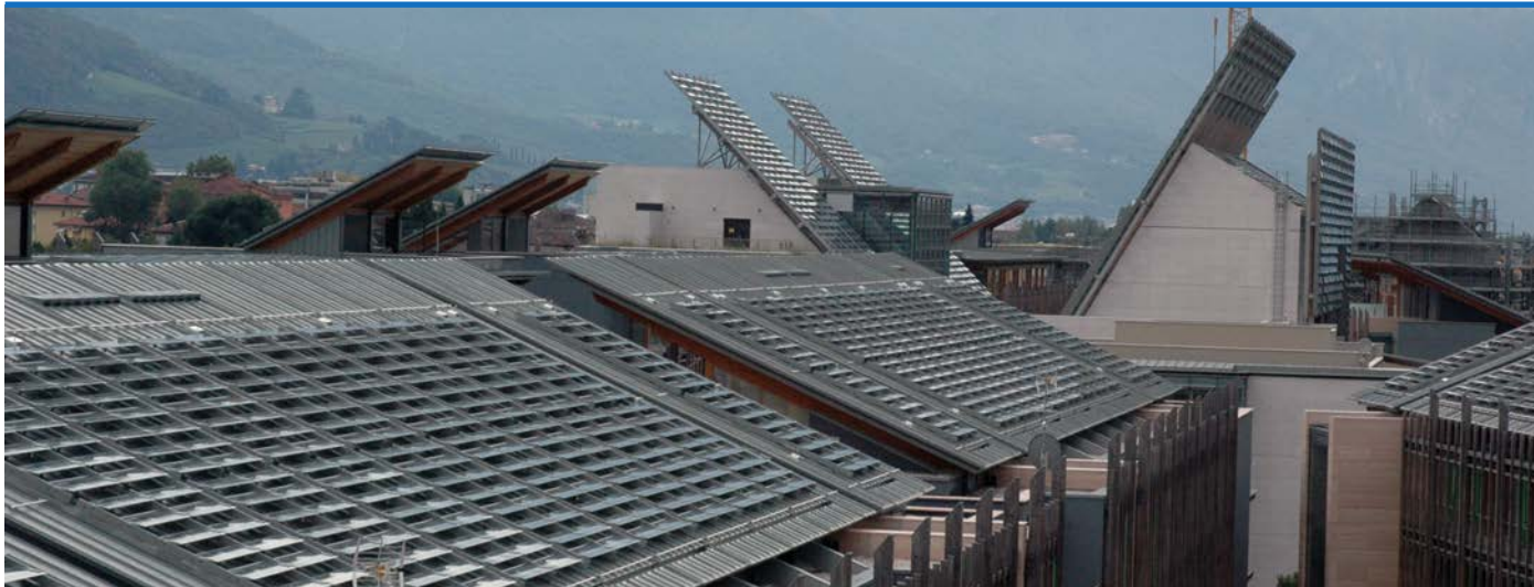
Figure 6 - System geometry: view of the PV systems integrated in the roofs from the terrace of the MuSe (Photo: © Silvia Croce).
