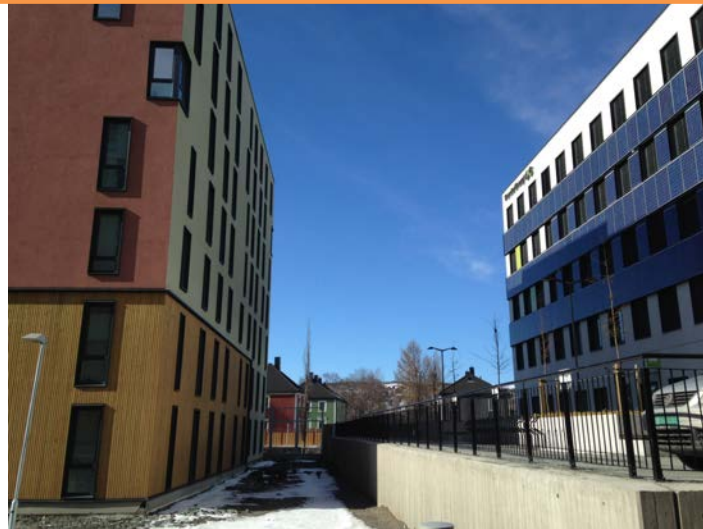
Figure 5 - A view of PV system installed on the South façade of the building shaded by the student block in front of it. (Photo: © Carmel Lindkvist)
