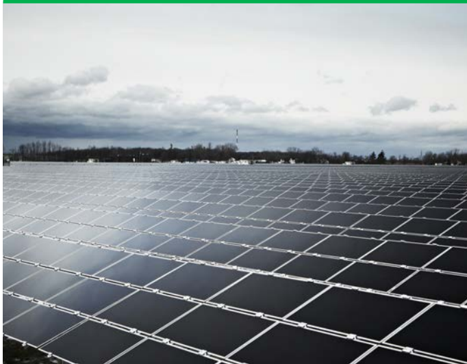
Figure 7 - Solar Panels. (Source: © Enbridge Inc.)
