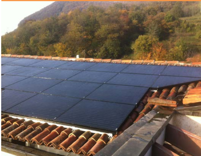
Figure 1 - View of the PV panels installed on the roof of one of the house in the Castel San Pietro (Photo: © SUPSI)
