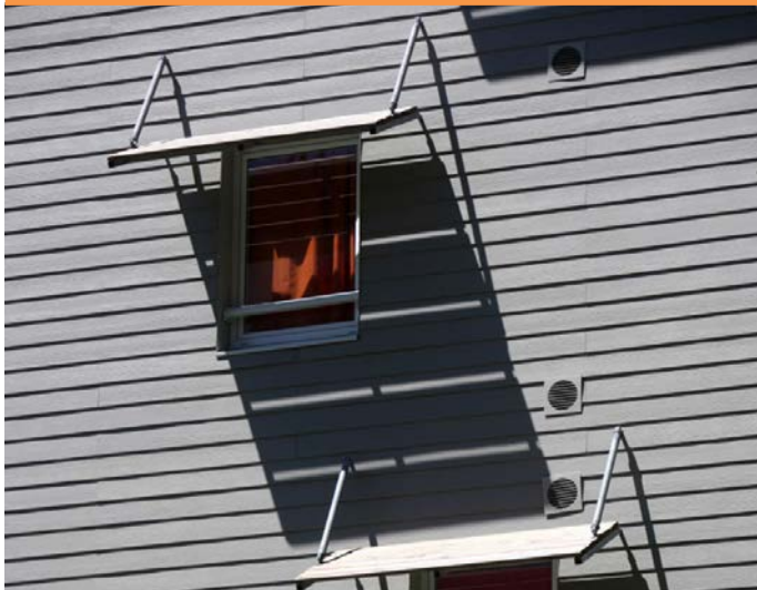
Figure 4 - Various solar shading devices, optimised according to the orientation of the facades, protect the numerous openings. (Source: © H. Douris).
