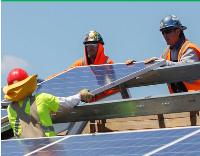
Figure 11 - Installing solar panels. (Source: © Postmedia Network)
