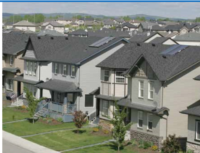
Figure 2 - DHW PV panels visible on front sides (Source: © CanmetENERGY, Natural Resources Canada)
