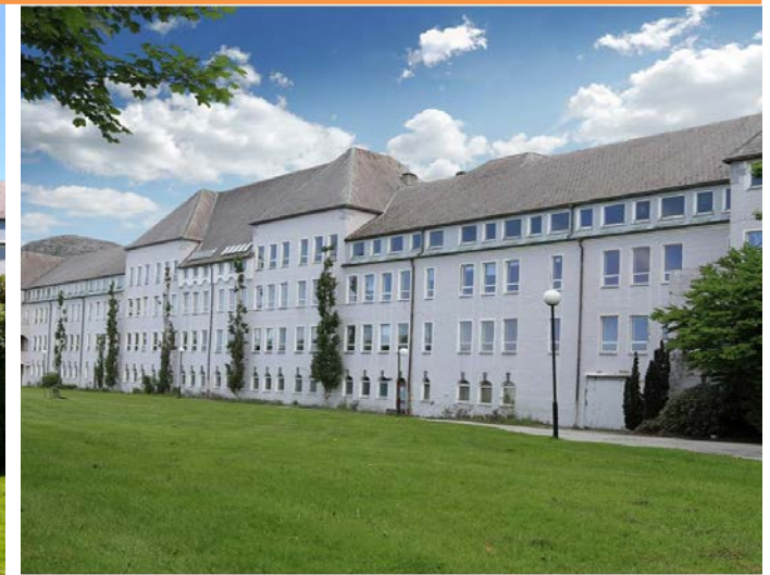
Figure 2 - West view of the main building of Dale – Protected mental institute. (Source: © KOKO architects)
