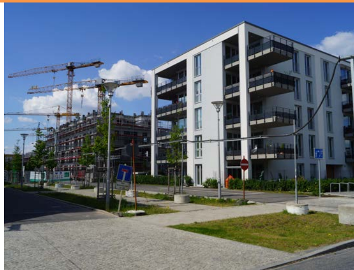
Figure 33 - Construction site for residential buildings. (Photo: © Margarethe Korolkow)
