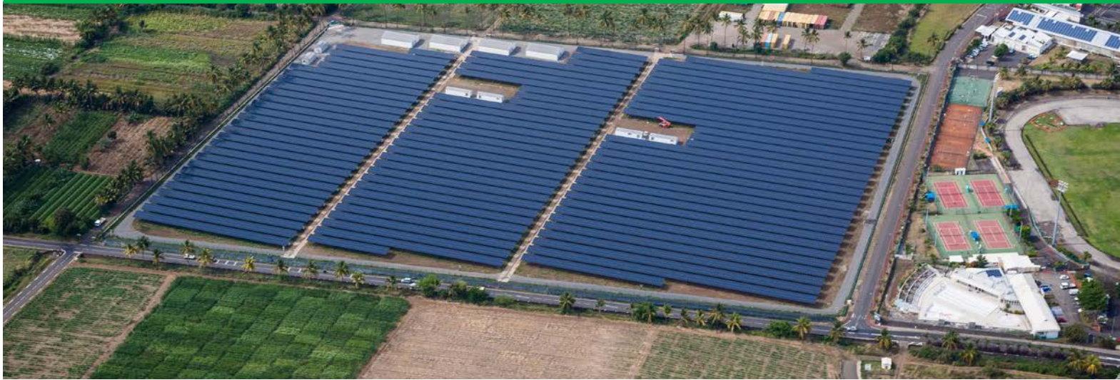
Figure 7 - Aerial view of the Agrinergie 5 from the North-East (Source: © akuoenergy.com)
