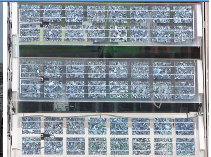
Figure 7 - System materiality: glass-glass PV modules installed on the façades (Photo: © Silvia Croce)
