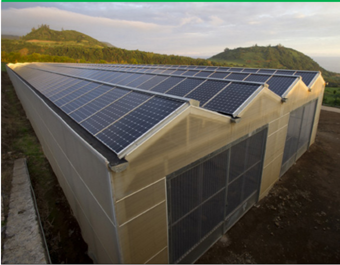
Figure 12 - Detailed view of the PV system integrated in the roof of one greenhouse block. (Source: © akuoenergy)
